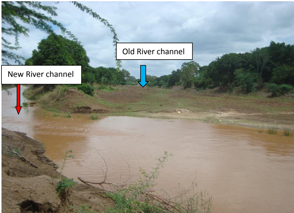
Plate 1: River Tana channel diversion at Mnazini area near Garsen town
